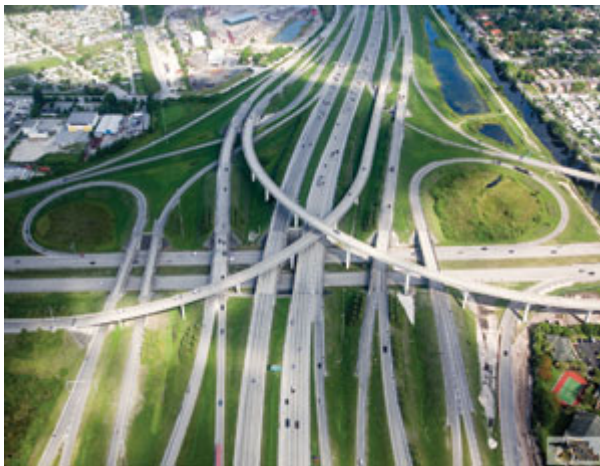
Photo Courtesy Of The Corridino Group The I-595 expansion deal, including new managed lanes, was tough to close.
